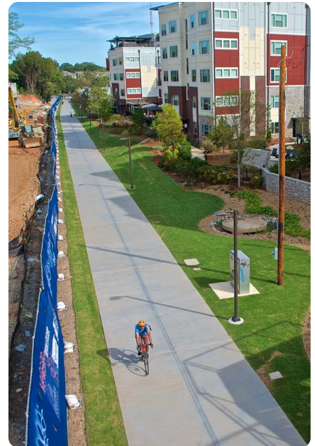
Fig. 19: View of the BeltLine in Atlanta, Georgia.
