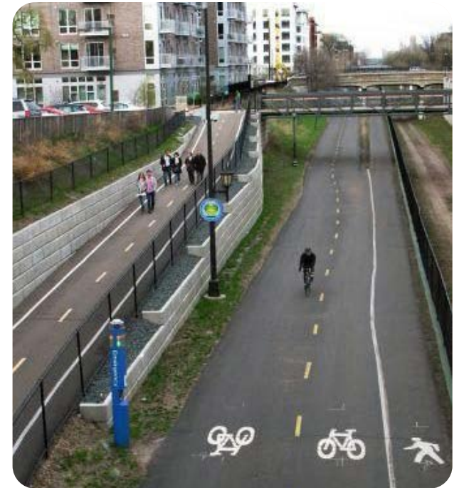
Fig. 52: Extending the Midtown Greenway would create stronger connections among the region's commercial districts and neighborhoods.
