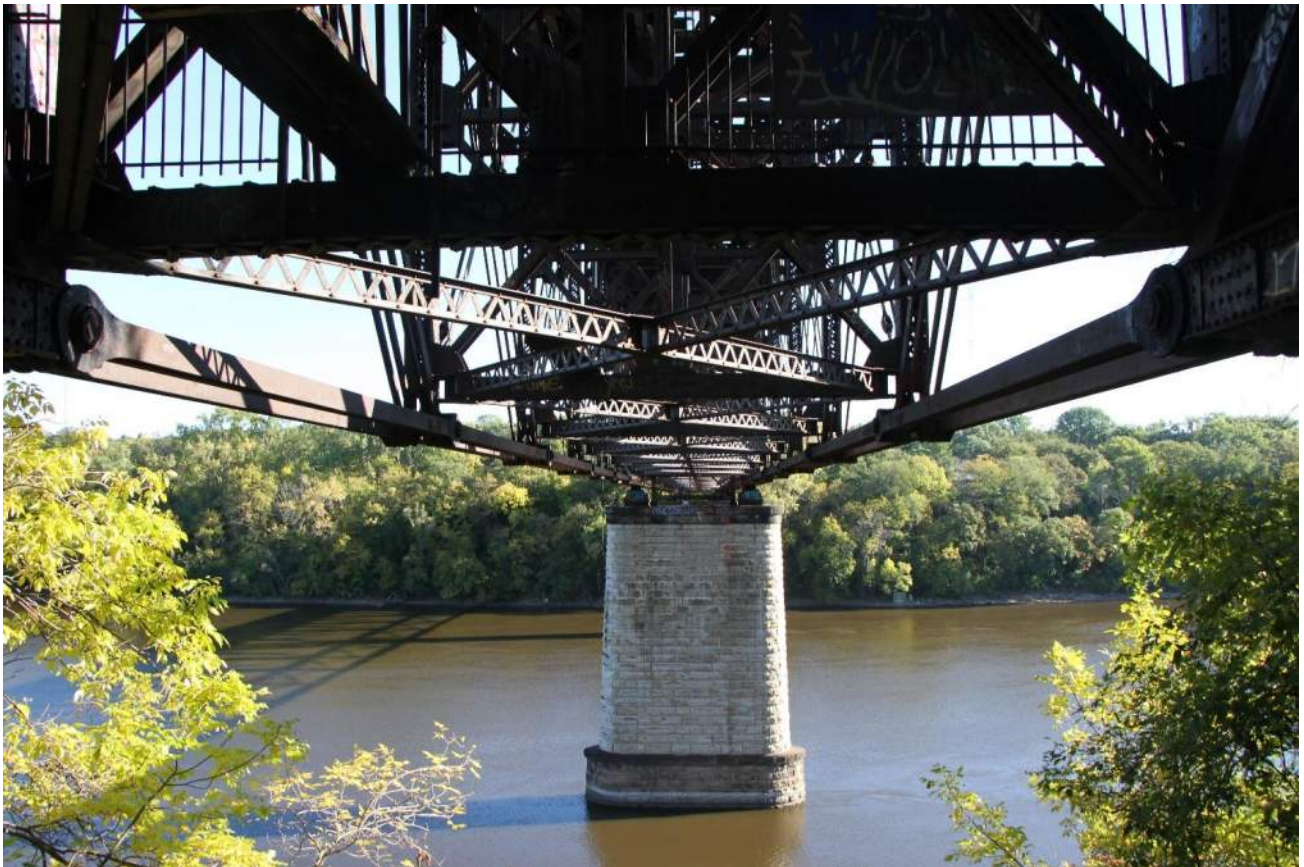
Exhibit B6: West river pier and underside of Span 2 looking east
