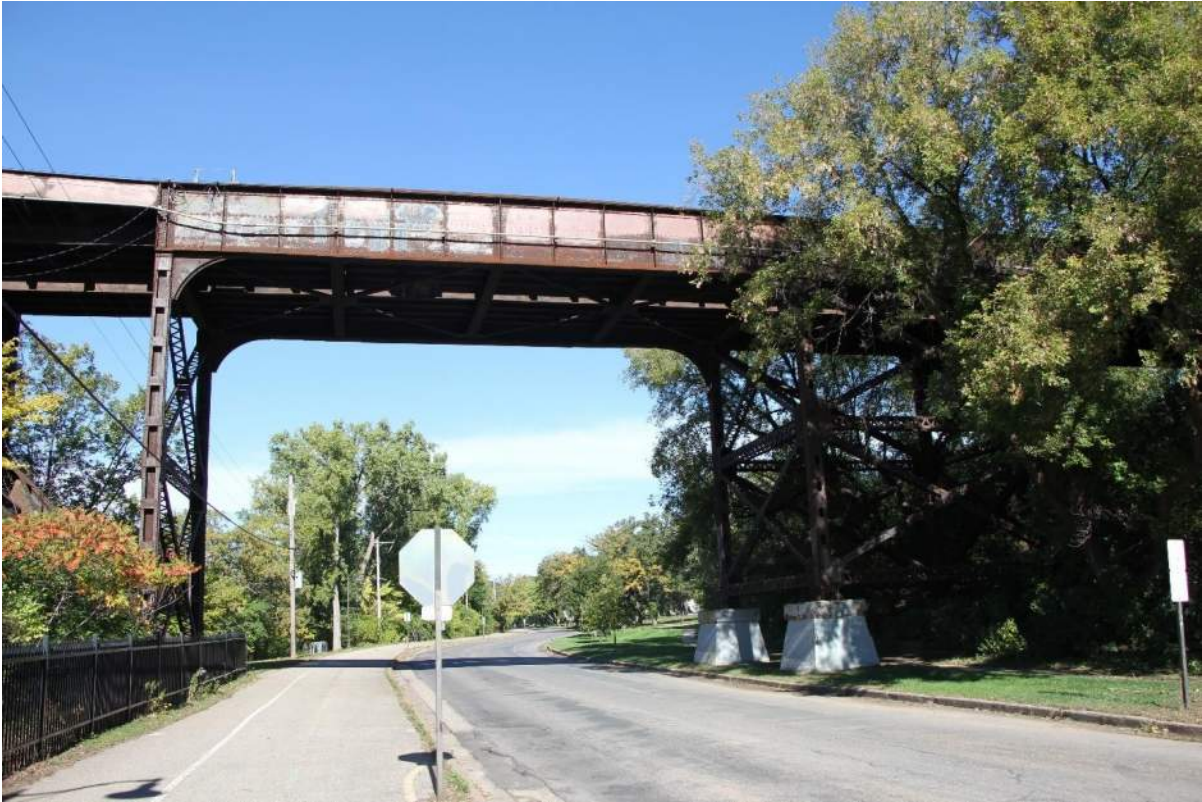
Figure 7: Span 5 looking north over East River Road, Span 6 obscured by vegetation
