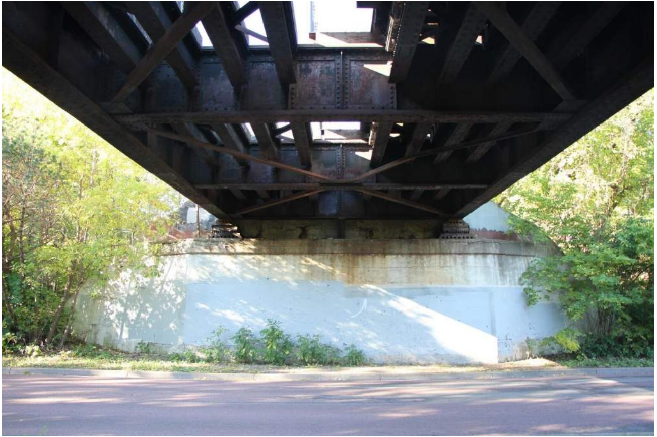
Exhibit B5: West Abutment and underside of Span 1 looking west
