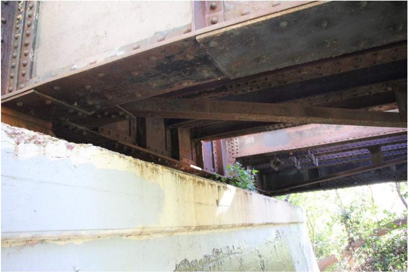
Exhibit B7: East Abutment looking southeast
